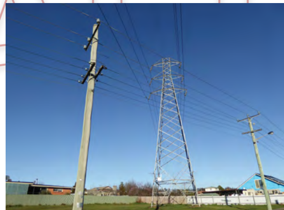
Open space encumbered by an electricity pylon, Youngtown
